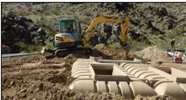
Big equipment necessary for this work
