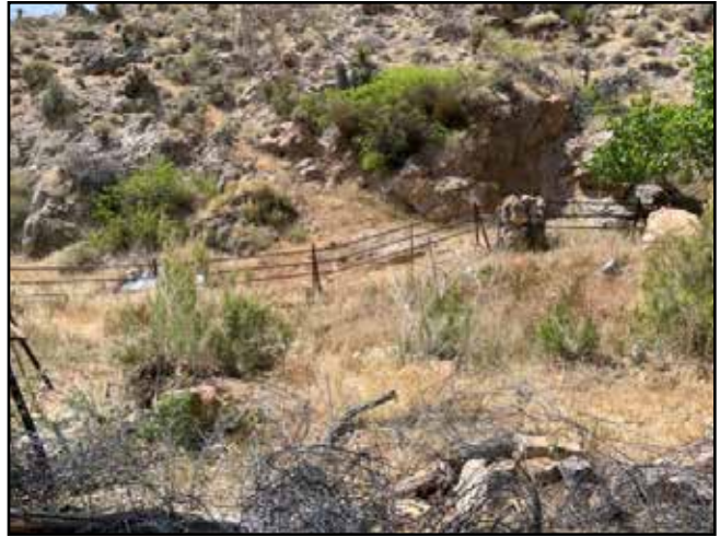
The new jack rail fence at Crystal Springs in the Kingston Mountains
