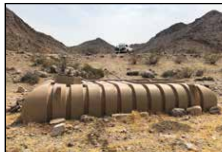
100' of hose stretched while 275-gallons of water is fed in to the 2300-gallon temporary tank.
