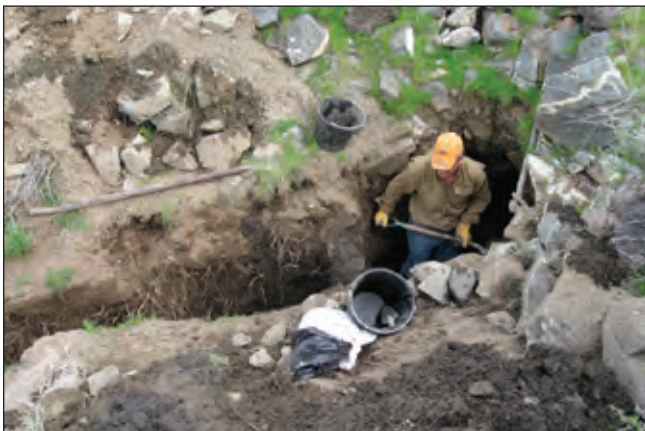
Chuckwalla Spring, end of digging in March, note concrete above Neal's shoulder
