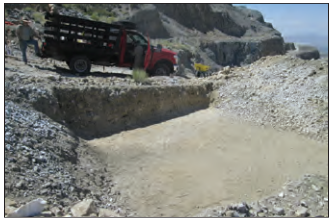
Mitsubishi Mine, hole ready for tanks (now it has some fines)
