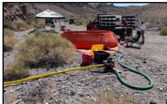
Above: Big Red dropping second load of water to the 3000-gallon bladder tank as the Mark 3 Wajax Water Pump begins operation..
