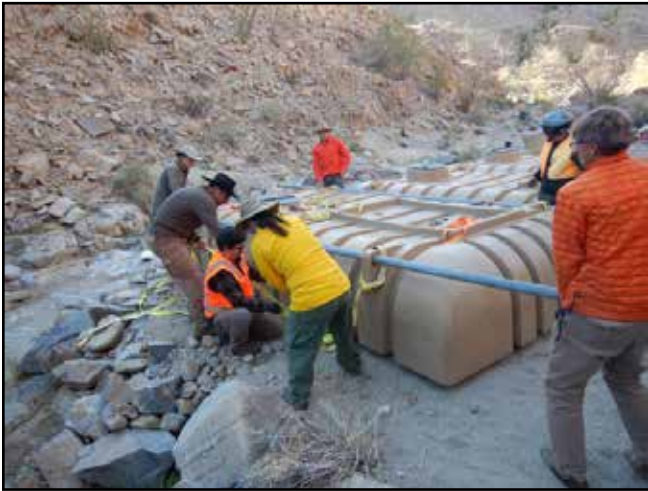
Tank being positioned
