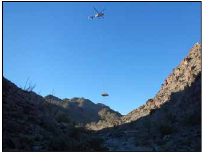
One of the new tanks being airlifted in
