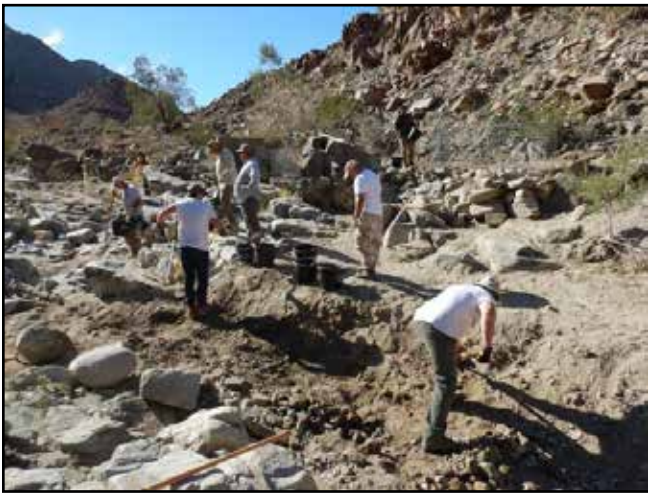
Next step: building the pad
