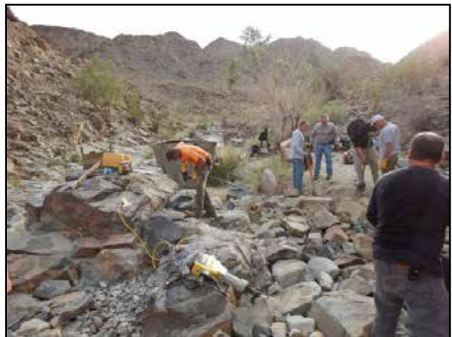
Work begins with rock removal - some huge ones!
