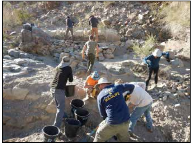
Building rock gabions
